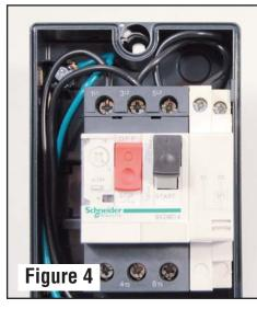
**IMPORTANT** Be sure that the switches and motor starter are <u>all the way to</u> <u>the right</u> when reassembling. This will allow switches to align with cover.
