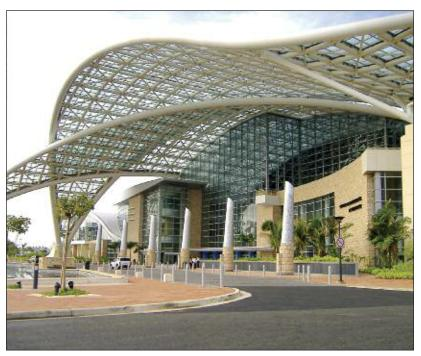
Puerto Rico Convention Center San Juan, PR U.S. Aluminum Hurricane (Impact) Resistant Systems are constructed to provide essential protection in regions where impact resistant glazing systems are mandated. These systems have passed the stringent requirements of the Miami/Dade County protocols for protection from high winds and wind-borne debris.
