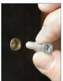
Lastly, insert the screw or bolt into the Rivet-Nut and tighten. The door stile is now ready to receive a Push/Pull Handle.
