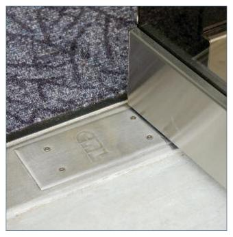
These Narrow Width Floor Mounted Door Closers are preferred on doors installed with Patch Hardware because smaller cover plates are more attractive in this type of installation. The Door Closer has separate valves to control closing and latching speeds. 90 Degree Hold Open and No Hold Open models are available.
