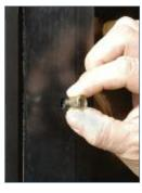
Second, insert the Rivet-Nut into the hole until the collar on the Rivet-Nut is against the door's stile
