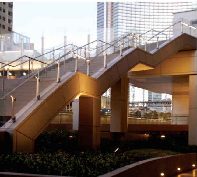
Custom Fabricated Stainless Steel LED Lighted Railing and Hand Rail System
