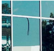
Vinyl side load gaskets can fall out. USAL uses Top-Loading E.P.D.M. Gaskets.
